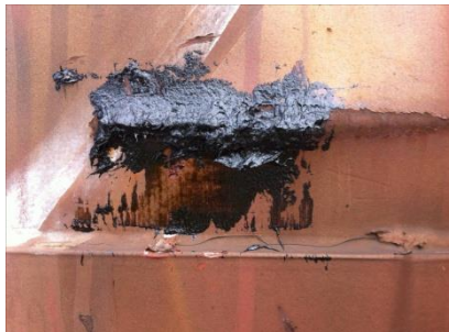
Roofing cement repair
