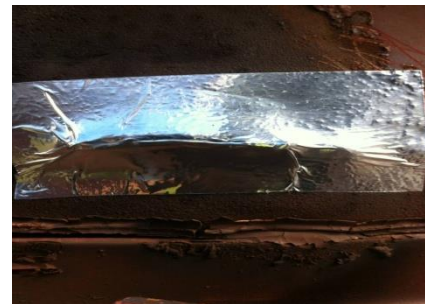
Silver/rubber seam tape repair
