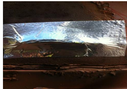
Silver/rubber seam tape repair
