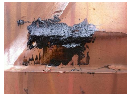
Roofing cement repair
